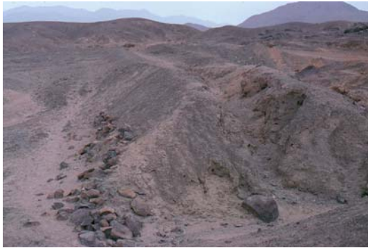
Water Management in Peru. Fig. 5 View of the cross-section of the Hoya Hondada aqueduct at the destroyed south end; height of the channel approximately 5 m from ground level. Photo by C. R. Ortloff.
